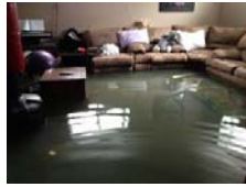
Floods (not leaks)
